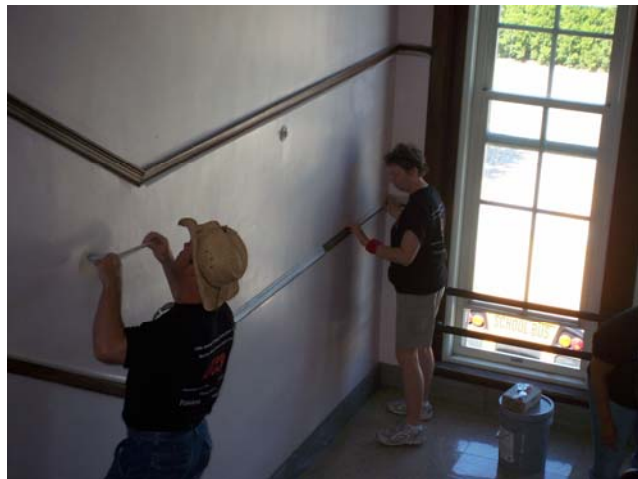
Painting prep at Bateman Elementary.
